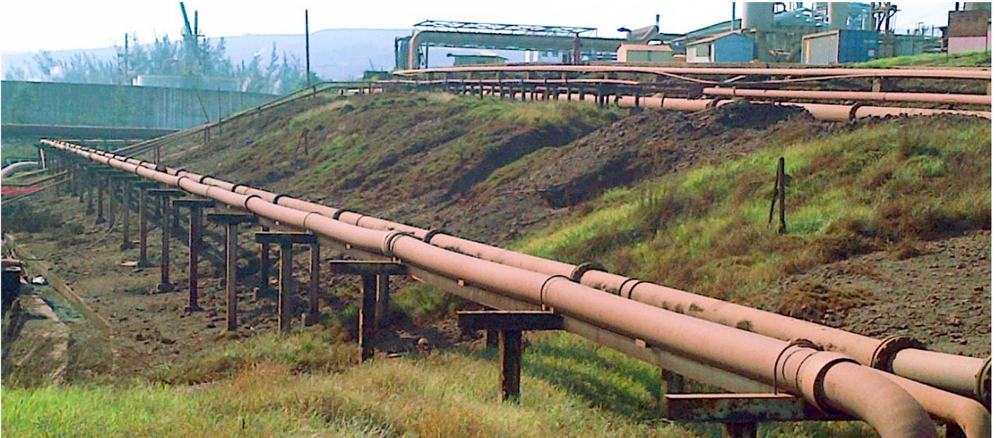
Transportation of mixed liquid and corrosive vapor (H<sub>2</sub>S) from the dehumidifiers
