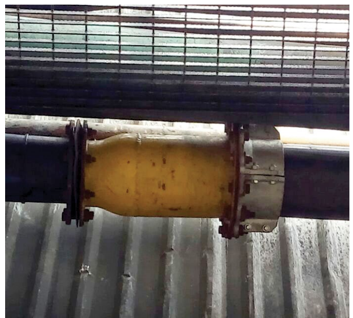
Transition from Pexgol 10" to an existent coated steel 10"x8" reducer
