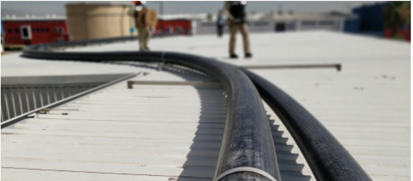
Water transport from a borehole with low pH.
