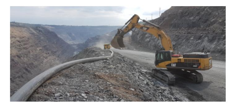
Installation of Pexgol pipes for drainage in a vertical ground
