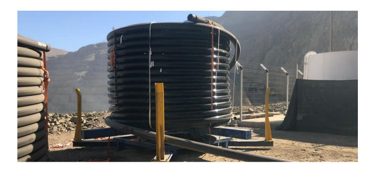
Installation of 3000 meters of PE-X pipe for an underground mine.
