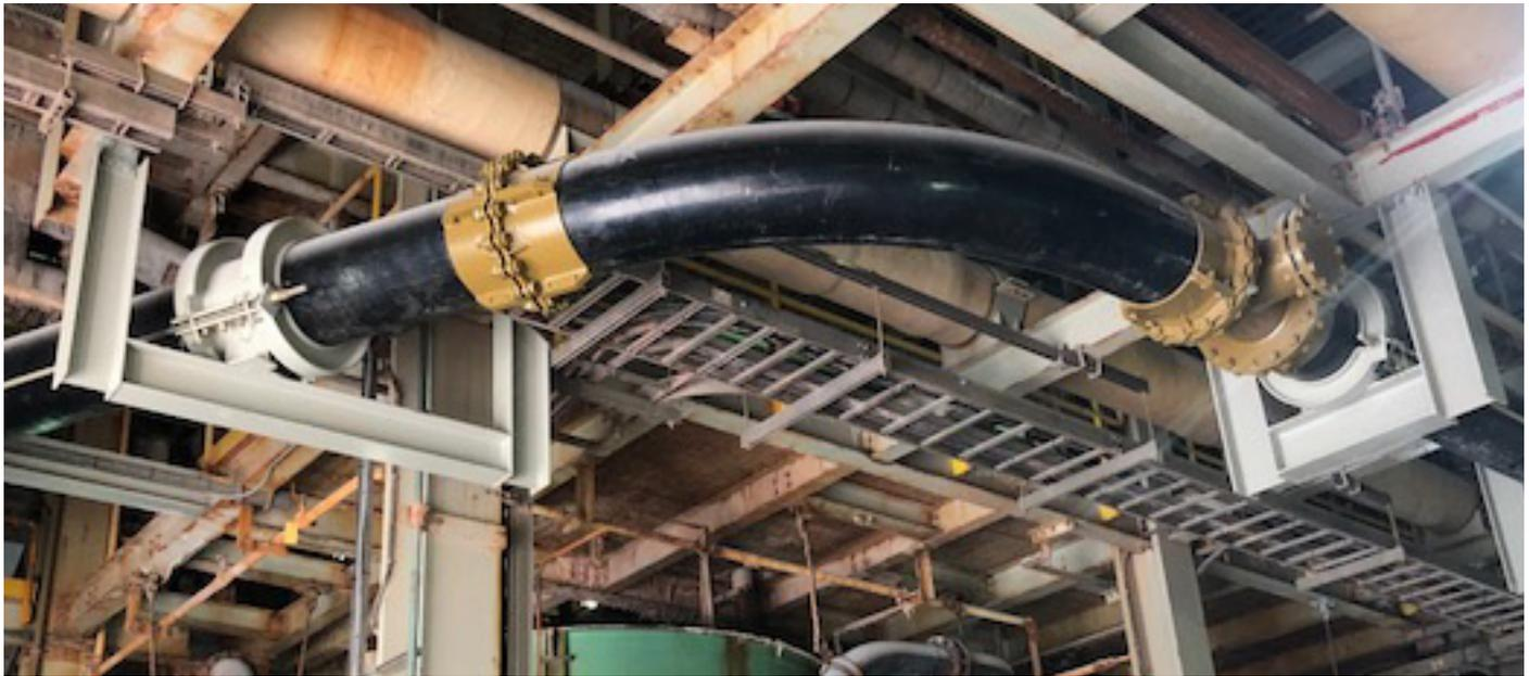
Installation of Pexgol pipe for a intake line to transport hot abrasive brine slurries.
